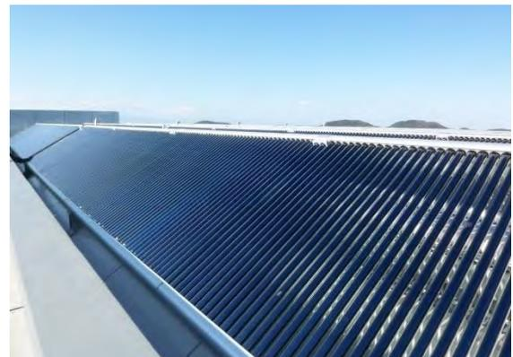
Fig. 7 EVACUATED TUBE COLLECTOR
