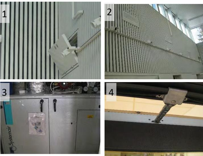
**Fig. 11** 1) HATCH SEPARATING RØDHETTE AND AGORA. 2) WINDOWS IN THE AGORA + INLETS FOR MECHANICAL VENTILATION 3) AHU 4) WINDOW OPENING CHAIN
