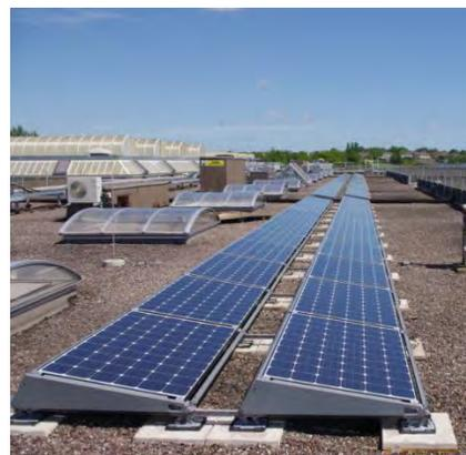
Fig. 7 INSTALLED PV ARRAY ON ROOF OF EXISTING BUILDING
