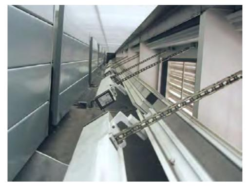
Fig. 10 INLET BOTTOM HUNG WINDOW AT THE BOTTOM OF THE CURTAIN WALL
