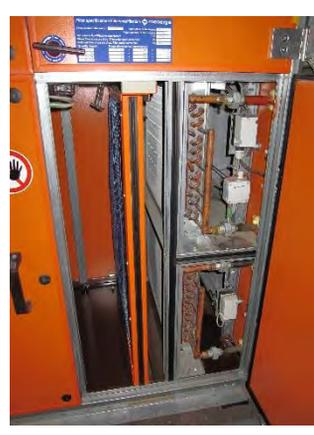
Fig. 7 HEATING COILS IN THE AIR HANDLING UNIT
