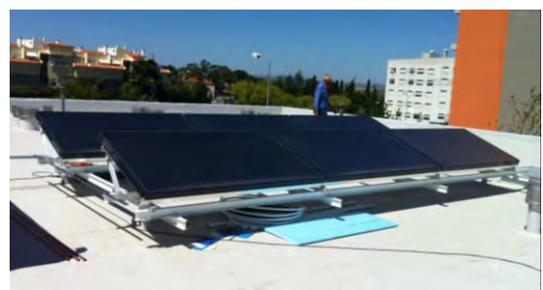
Fig. 5 INSTALLED ST PANELS ON CML KINDERGARTEN ROOF.
