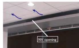
\*Slits are also provided at the ceiling to allow the air to flow into the centre void through plenum space.
