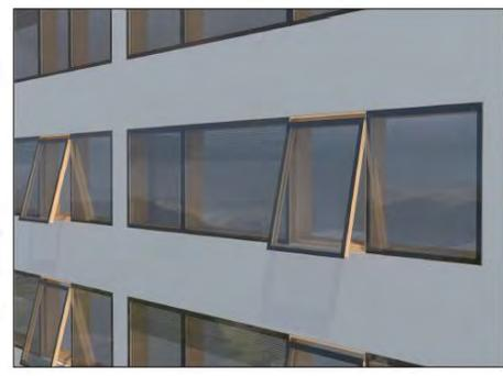
Fig. 9 CUSTOM-MADE TOP-HUNG PROJECTING-OUT WINDOWS, SOURCE: PASSIVHAUS INSTITUT
