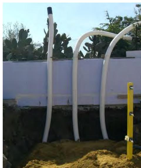
Fig. 8 EAHE AND MONITORING SENSORS INSTALLATION IN THE CONSTRUCTION SITE
