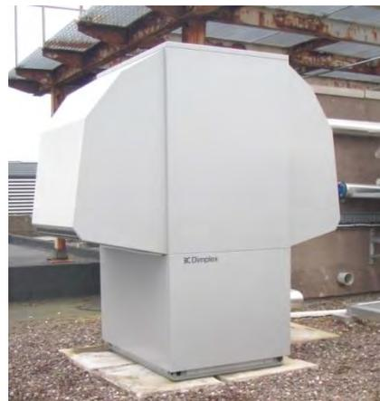
Fig. 5 AIR SOURCE HEAT PUMP ON ROOF OF ZERO2020 BUILDING
