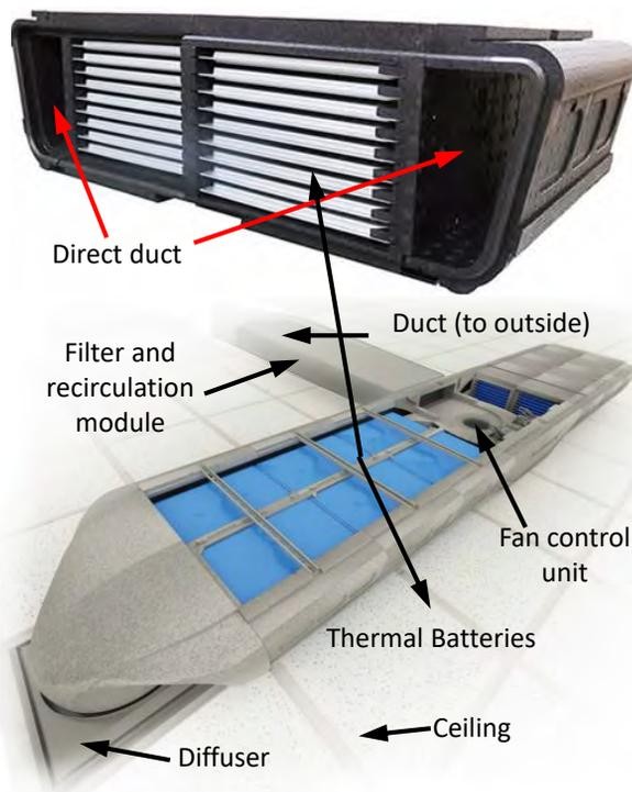
Fig. 5 COOLPHASE UNIT COMPONENT [4]
