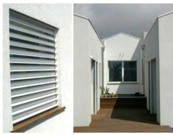
**Fig. 9** OPENABLE WINDOWS WITH AUTOMATIC EXTERNAL BLINDS AND THE EXTERNAL PATIO
