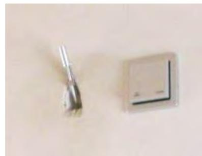
**Fig. 17** EXAMPLE OF INDOOR SENSOR INSTALLED TO MEASURE TEMPERATURE, RH, CO2 CONCENTRATION
