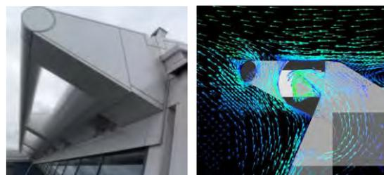
**Fig. 23** DETAIL DESIGN STAGE SIMULATION: AIR FLOW OF EXHAUST OPENING
