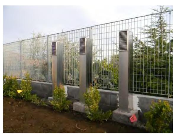
**Fig. 10** INLET DUCTS OF THE EAHE
