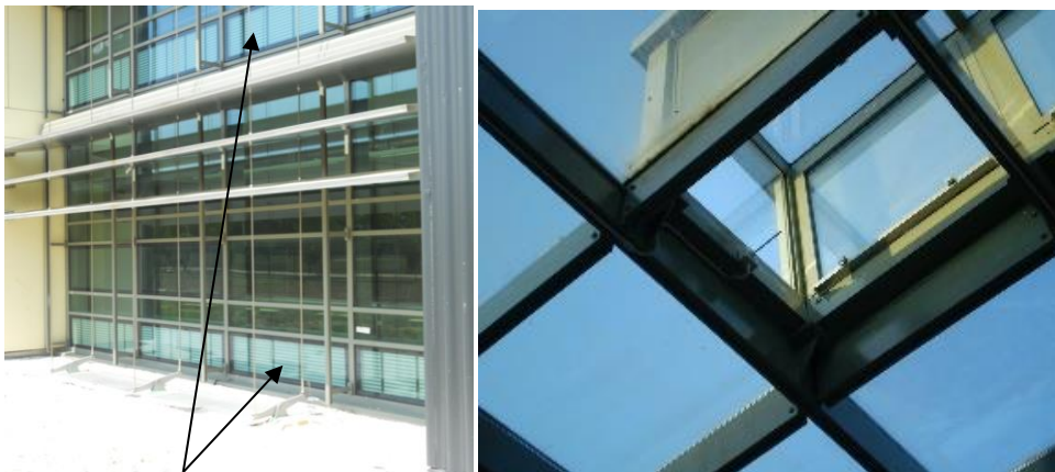
Image 04: inlet airvents - © G.Chiesa
