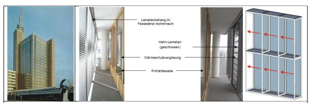
Figure 5.37. Double-skin high-rise office building Deutsche Messe Hannover, Arch. Herzog & Partner, Munich. Double-skin corridor façade. 1,32 m deep, double pane insulating glass in both façade layers, venetian blinds in between, openable windows in the inner skin, ventilation louvres in the outer skin.
