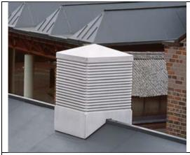
Figure 5.32. Modern bi-directional windcatcher with option for ducted air dispersal by Passivent, UK. Source:
