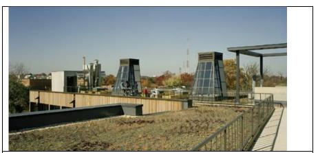
Figure 5.12. Solar ventilation chimneys, Sidwell Friends School, Washington D.C., USA. Addition and extensive renovation finished in 2008. Designed by Kieran Timberlake Associates. Source: www.solaripedia.com (29.12.2014).
