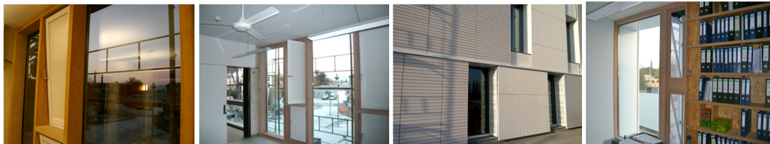
Figure 10: Tilted north façade vent, north façade open right, south window from outside, south vent from inside
