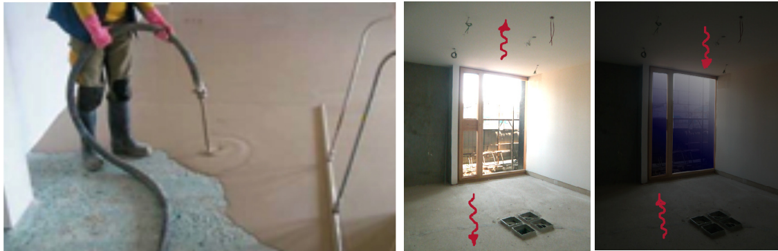
Figure 5: Floor and ceiling are composed by massive materials with high thermal mass
