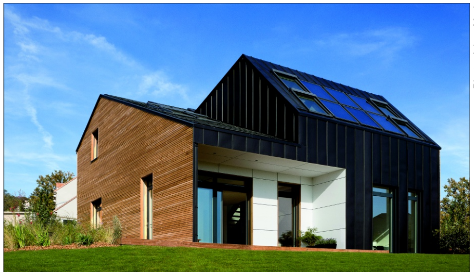
AN EXAMPLE OF REAL PRACTICE Maison Air et Lumière in Paris, France: A one-family house designed to avoid overheating through the use of advanced ventilative cooling and solar shading strategies.
