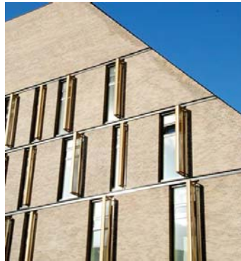
Court building Mechanical- and natural ventilation depending on the area.
