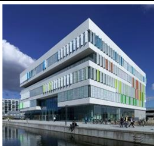
Image 01: South and west façade ©Adam Mørk
